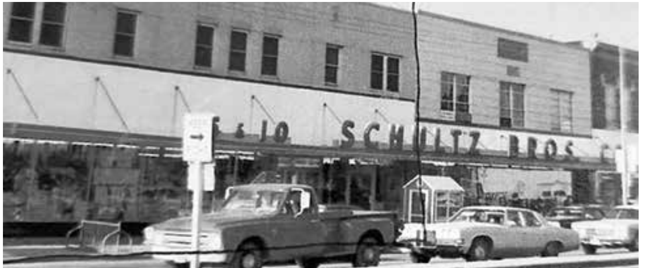
500 block of South State Street in the 1970s
