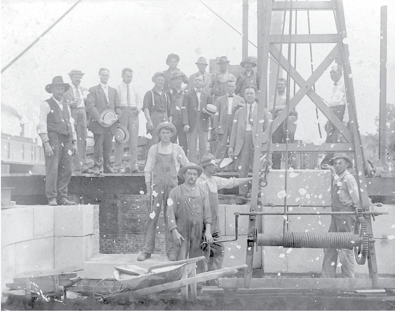
Construction workers and Post Office staff pause work for a photograph taken around the mechanism used to set large granite blocks for the construction of the Belvidere Post Office around 1910. These blocks can be seen forming the foundation of the building today.
