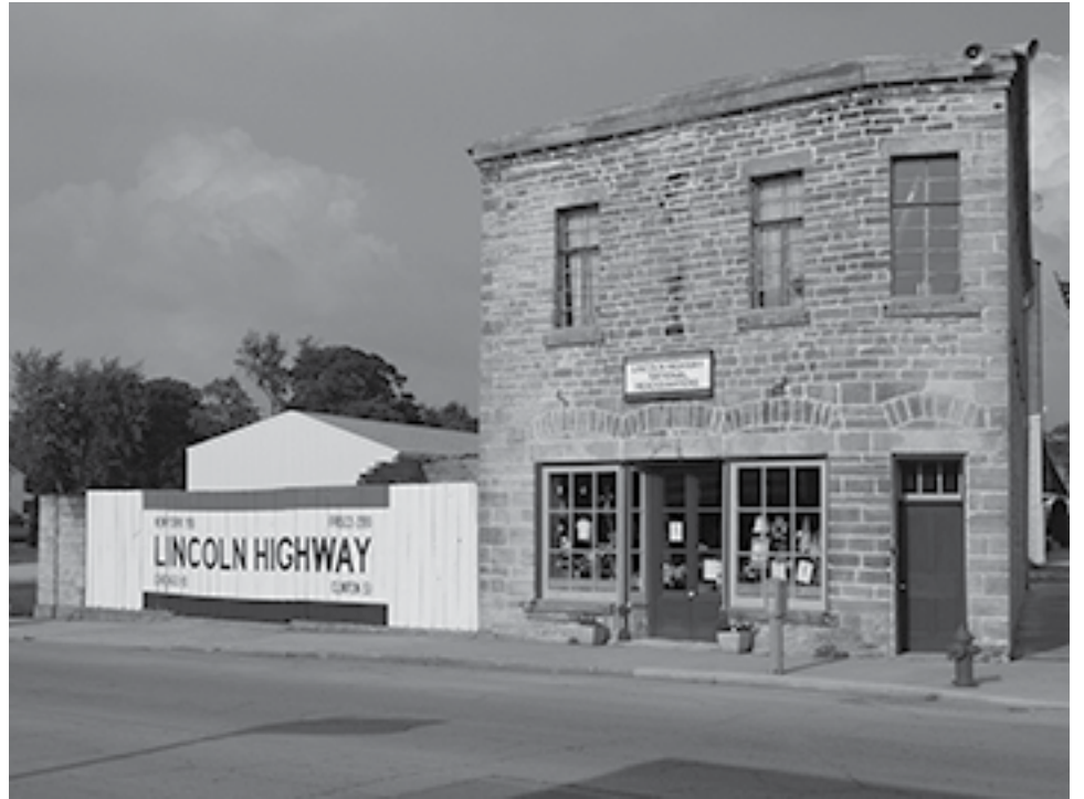
From 1860 to 2019 the H.I. Lincoln Building, now the Lincoln Highway Interpretive Center, has been a major feature of Franklin Grove’s business district.
