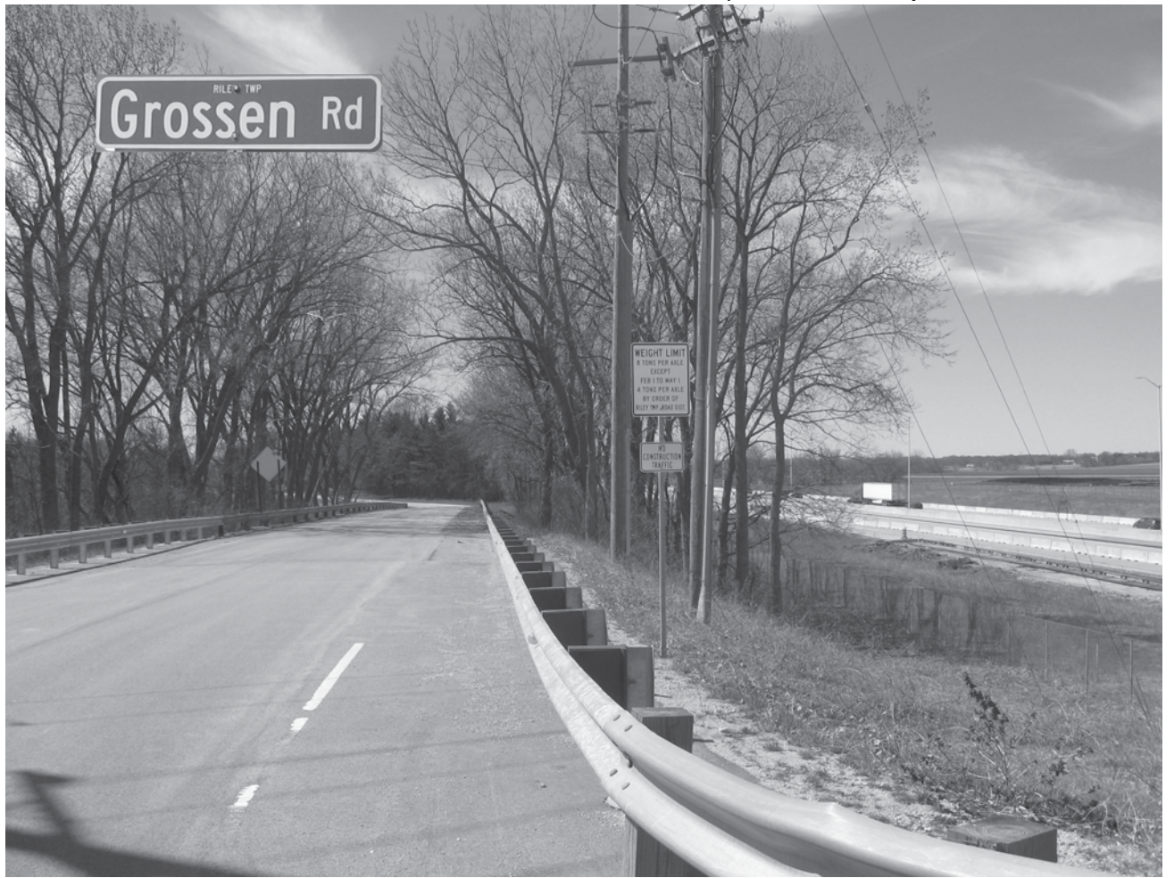
Grossen Rd. at Illinois 23, south of Interstate 90
