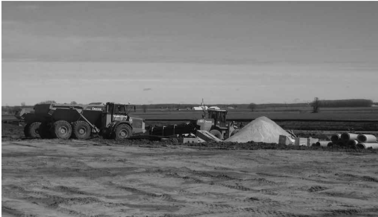
Construction along Illinois 23
